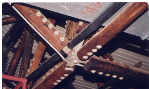
Fig 1. Common SDT connection method.
